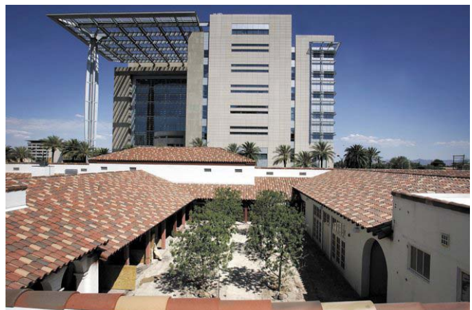
The Fifth Street School is set against the backdrop of the Lloyd D. George Federal District Courthouse in downtown Las Vegas. For Robert Dorgan, director of the Downtown Design Center, which will be housed in the renovated school, the contrast in architectural styles visible at a glance is intriguing.
