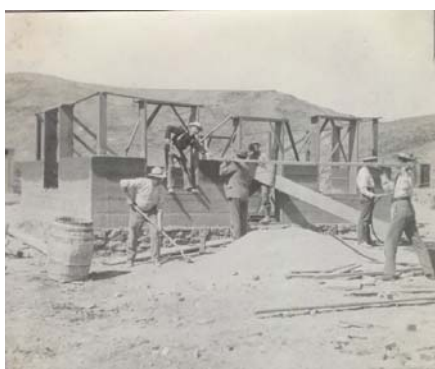
T. A. JOHNSON's residence in course of erection 1906
