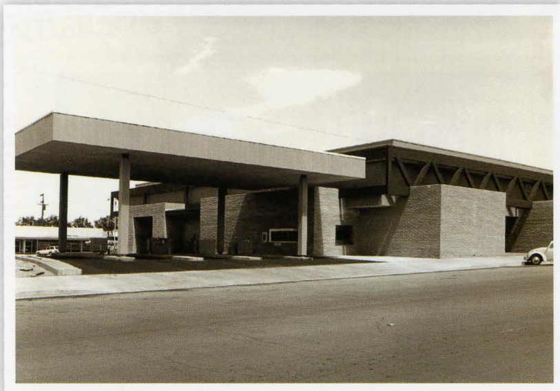
New Bank of Nevada building with drive-thru teller service.
