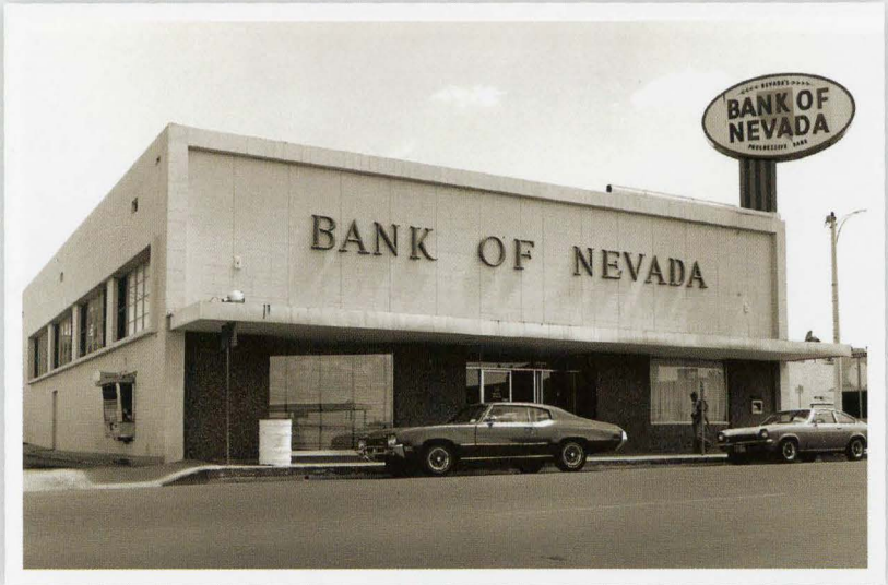
Original Bank of Nevada building in Henderson.
