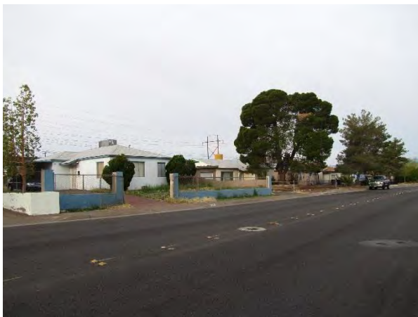
A neighborhood overview of the south side of Basic Road in Townsite.
