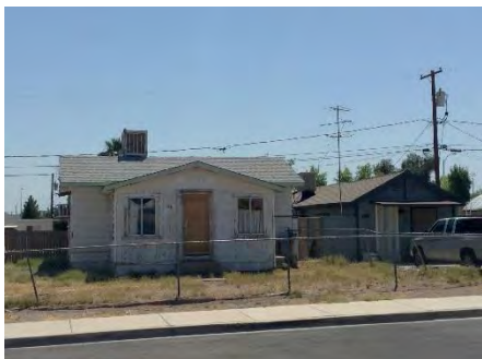
A sample property type of Townsite housing surveyed at 1816 Allen Avenue.
