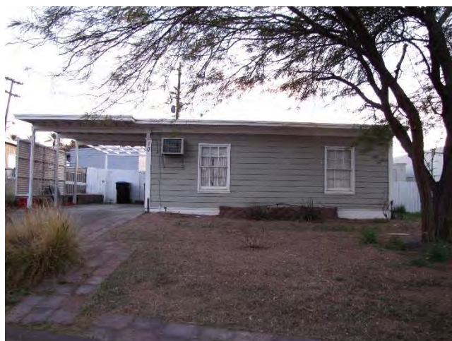
A typical original Townsite house at 10 Idaho Street.
