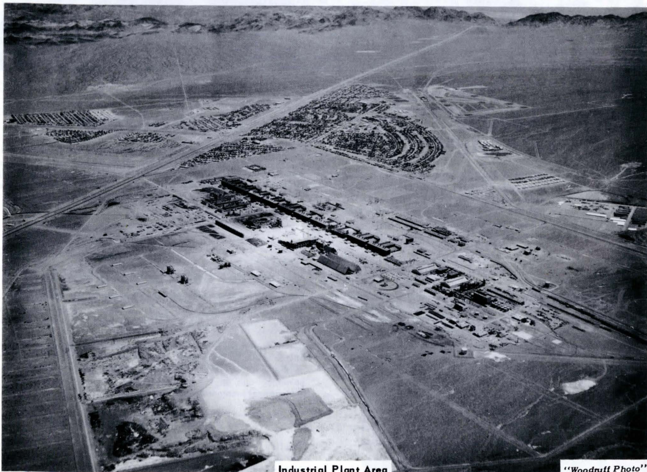
Industrial Plant Area
