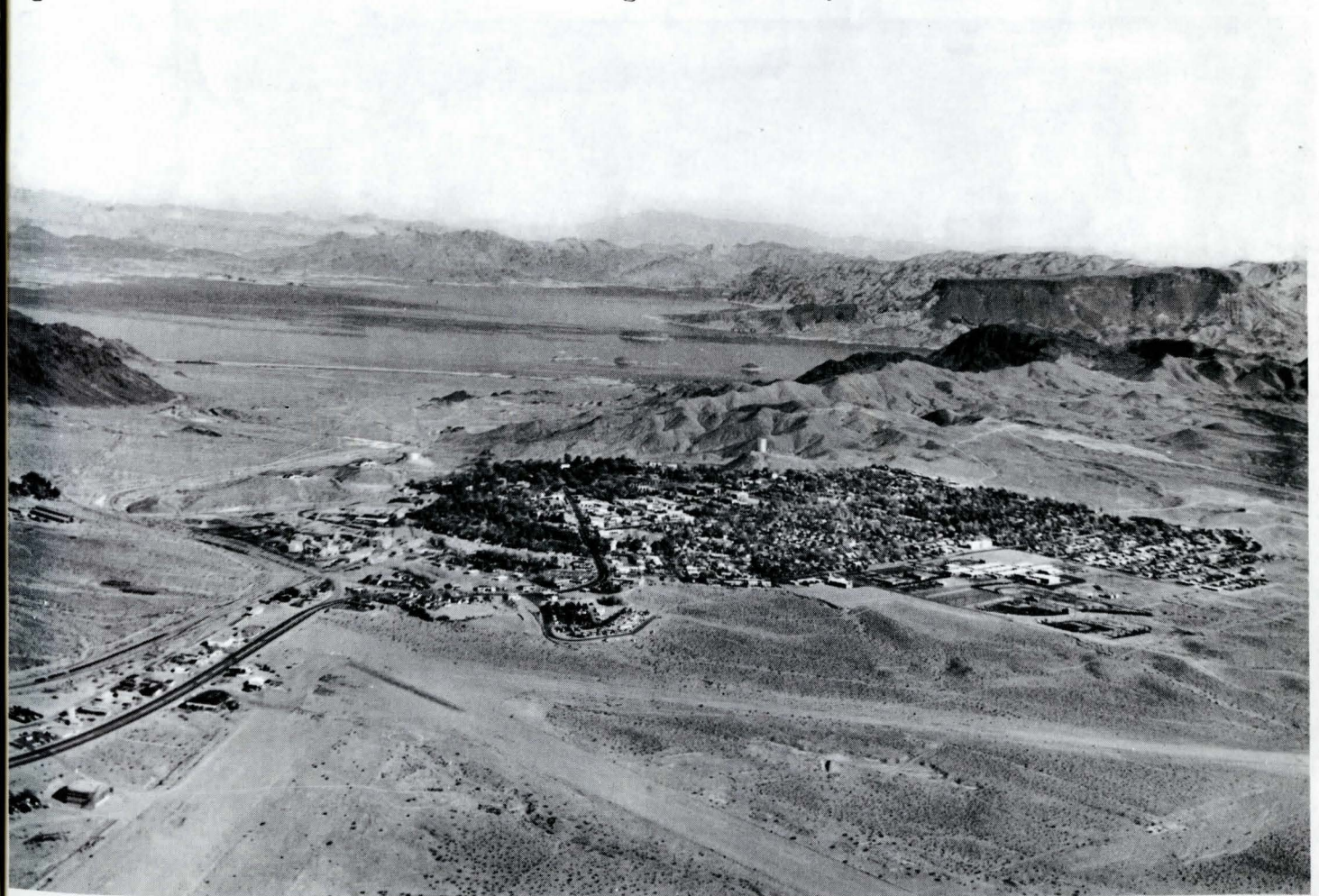
Photo Courtesy of Bureau of Reclamation
