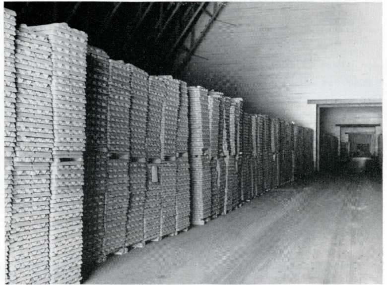
INTERIOR MAGNESIUM STORAGE BUILDING
