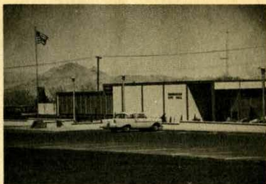
HENDERSON CITY HALL
