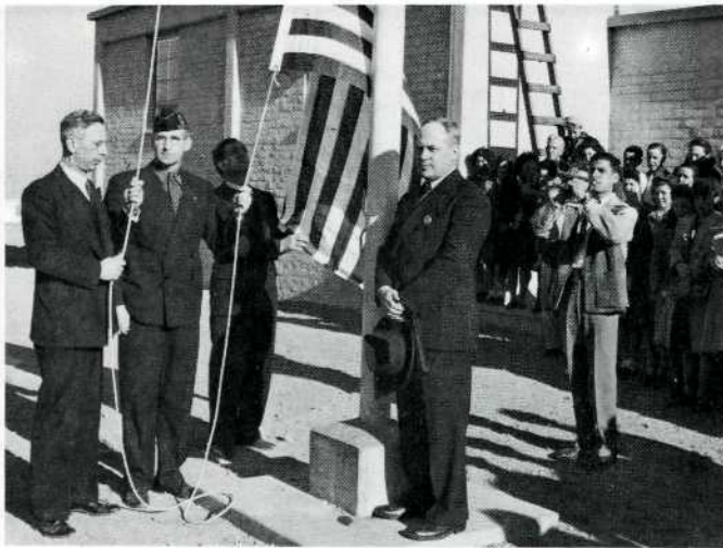
BASIC BOMBARDIER: Aug. 27, 1943—Construction of Henderson Postoffice Building, Townsite center, was begun the past week by O. J. Schrer Company for PDC, and is to be completed in about 75 days. The main structure will be 97 x 48 feet, concrete-block walls and concrete roof—one story with high ceiling.
