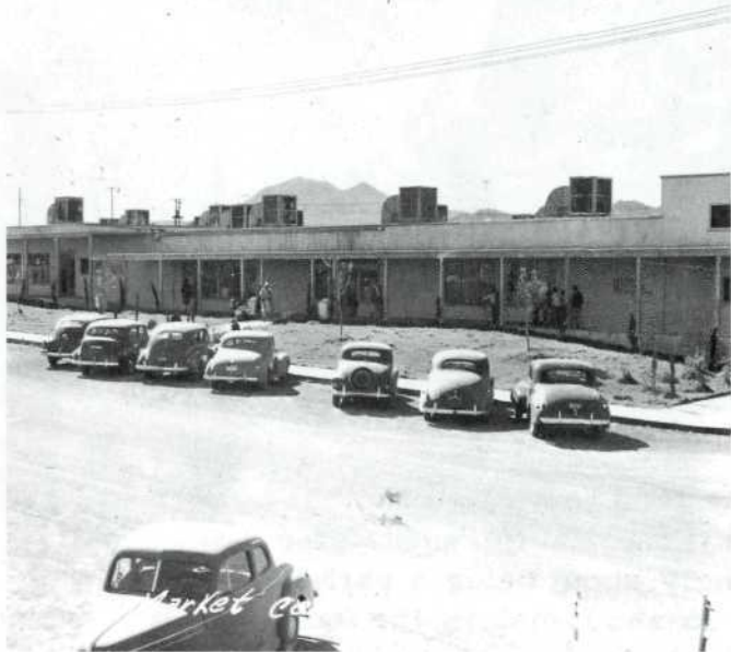
BASIC BOMBARDIER: Nov. 17, 1944—Portion of the Henderson shopping area in the townsite showing Nevada's largest grocery and market on the extreme left, department store and beauty shoppe on the corner. DPC Housing offices are on the second floor. Managing authority rests with Fred Unsworth, Housing Manager, and a staff of assistants. Information from store owners is that they will remain open as long as there are people in the community to serve. That holds good for the barber shop, theatre, recreation center, shoe repair shop, telegraph office and drug store. Disposition of houses—an even thousand of them—has not been decided by Washington Housing headquarters.
