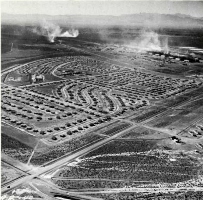
Aerial photograph of BMI taken September 15, 1943. Ventilators can be noted adorning the tops of all the metal units, relieving the unpleasant working conditions characteristic of early BMI operation.
