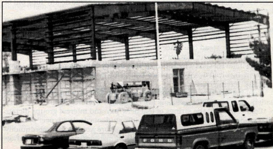
Rancho High School's new gym under construction
