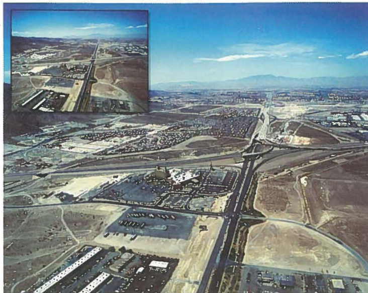
System to System interchange connecting I-215 to I-515/US 93- US 95, completing the southern beltway to full freeway standards
