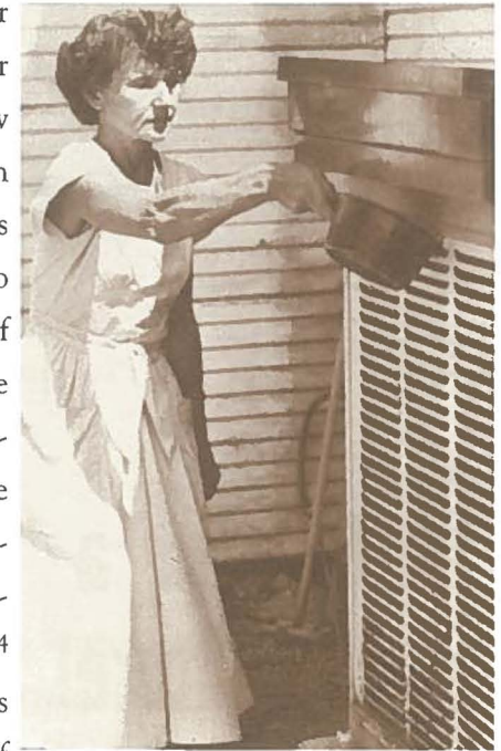
Resident hand pours water on cooler pads due to low water pressure, circa 1955
