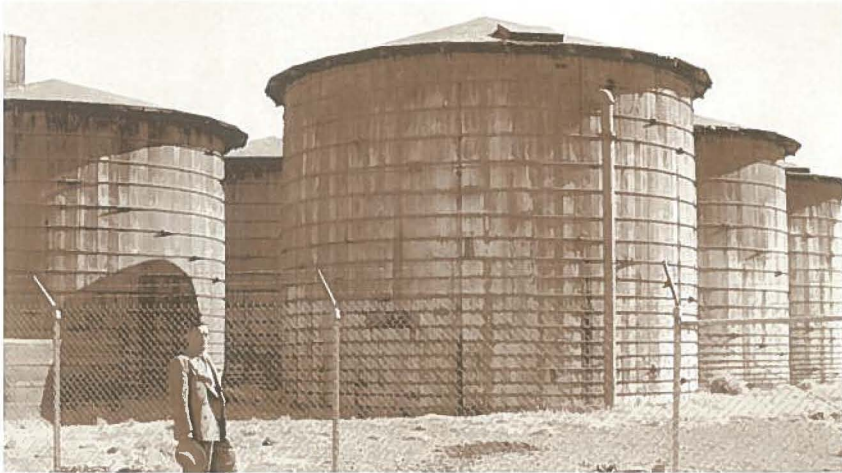
New water storage tanks located at the foot of Black Mountain, circa 1950's
