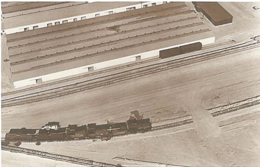
Eighteen miles of railroad track existed on the BMI plant site
