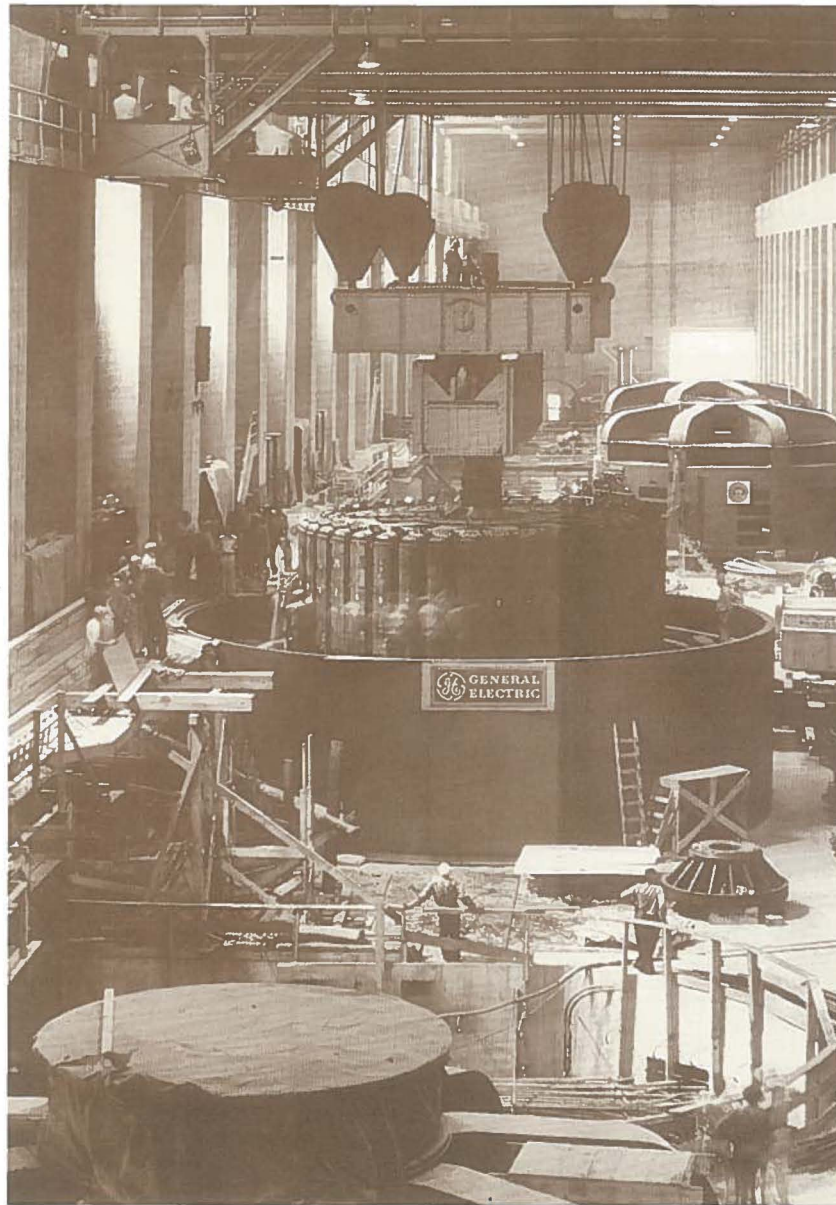
A five-hundred-ton rotating field of one of the largest generators in the world, Hoover Dam, July 31, 1936
