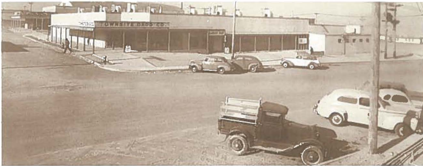
Townsite Drug Co., located on the corner of Market and Army Streets, circa 1940's
