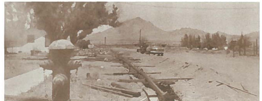
Installation of water lines to the residential area, circa 1950's
