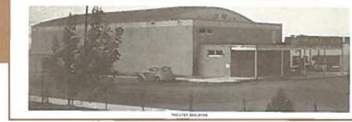
THE 5-STAR BUILDING Size: 40' x 110' Area: 22,000 sq. ft. Ceiling: 10-0 ft. h. Culding: 12' average Floor: One, plus a second-story penthouse bank Roofing: Asphalt Siding: Ply-boarded framing, composition coated Floor: Concrete Roofing: Asphalt Siding: Natural brick veneer, 1/2" rubber tile and dash. Exposed Partitions and fixtures: Full
