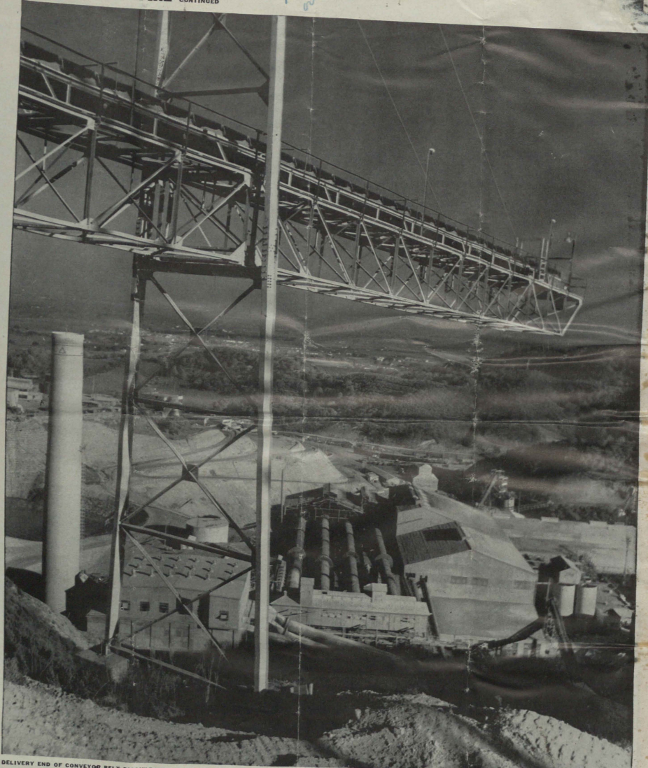
DELIVERY END OF CONVEYOR BELT DISCHARGES LIMESTONE ONTO PILE AT FOOT OF HILL. LIMESTONE WITH CLAY IS CALCINED BY NATURAL GAS IN FOUR ROTARY KILNS (CENTER)
