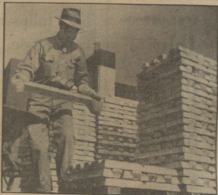
Here are magnesium ingots ready for shipment to defense plants. If the above ingot was composed of lead this workman wouldn't be handling it so easily. Its lightness—only two-thirds as heavy as aluminum—and strength are qualities that make magnesium so valuable in war production.
