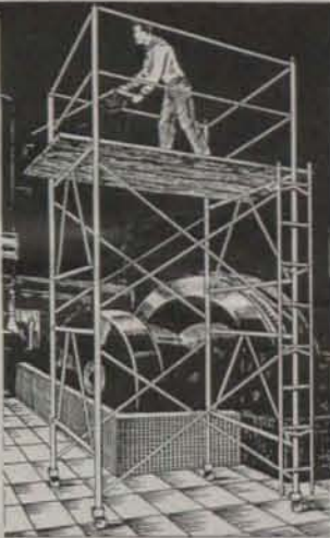
This 15 ft. rolling tower set up in 10 minutes
