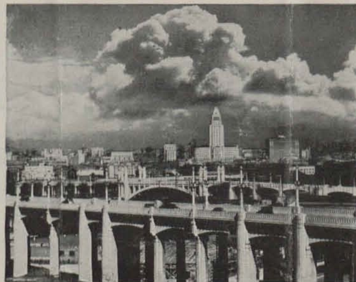
NEW CITY HALL'S tall tower rises above buildings of the Los Angeles civic center. Los Angeles River viaducts are in the foreground.
