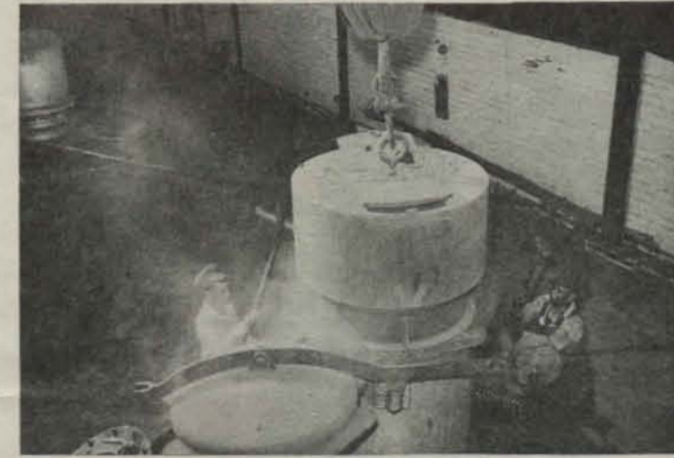
(Above)—This picture shows one of the chlorinators being charged. The pellets of raw material fall into great electric furnaces where chlorine gas is introduced and the magnesium oxide is transformed into magnesium chloride, then transported to the electrolytic cells, 880 of them, where metallic magnesium is recovered by means of electro-chemical action. (Below)—This ingot pouring machine receives the crucibles full of hot metal, tips automatically, and keeps the outpoured magnesium alloy flowing steady into moving molds. At the end they drop into bins—a finished product, ready for manufacture into implements of war.
