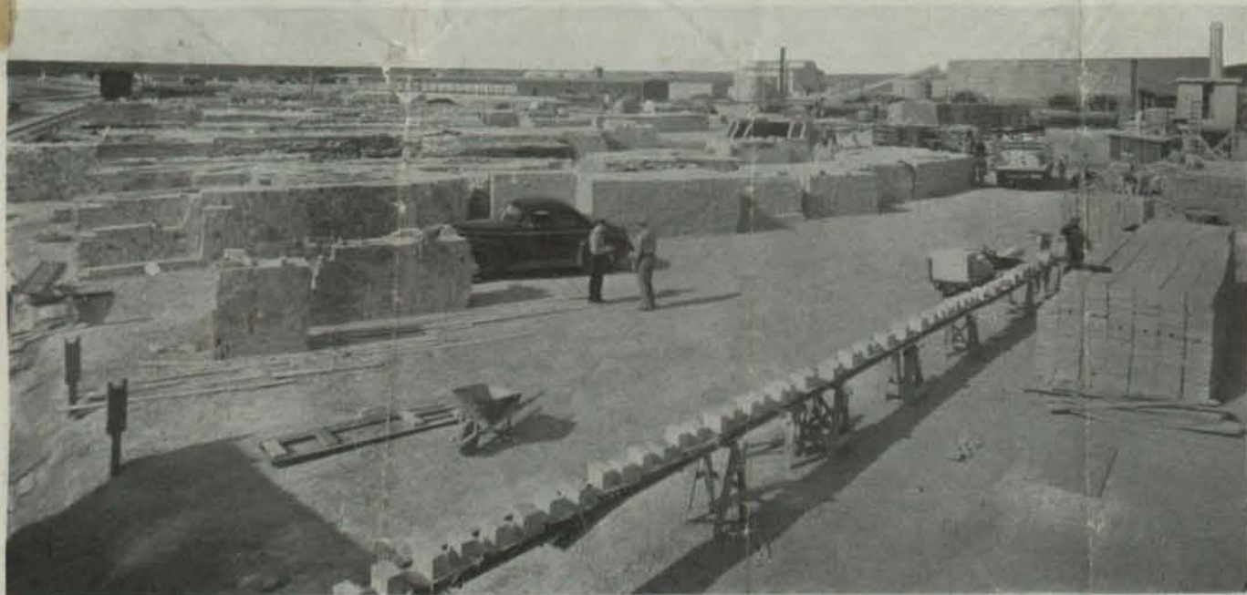
This is the stock yard for the many shaped firebrick which were used in the magnesium plant. A roll conveyor, shown in the foreground, carried brick on wood pallets by means of gravity.
