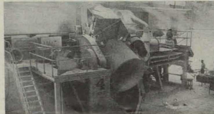
(Above)—This picture shows one of the chlorinators being charged. The pellets of raw material fall into great electric furnaces where chlorine gas is introduced and the magnesium oxide is transformed into magnesium chloride, then transported to the electrolytic cells, 880 of them, where metallic magnesium is recovered by means of electro-chemical action. (Below)—This ingot pouring machine receives the crucibles full of hot metal, tips automatically, and keeps the outpoured magnesium alloy flowing steady into moving molds. At the end they drop into bins—a finished product, ready for manufacture into implements of war.
