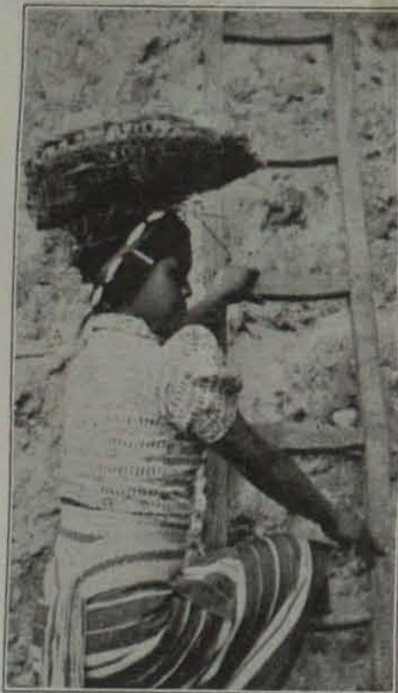
Igorot girl illustrating how ore was brought out of the Mankayan mine during the period of Spanish operation. The ore basket and ladder were found in old workings. The ladder still was serviceable when found although it had been abandoned in the stope nearly 70 years ago. The rungs were mortised into the side pieces and secured by wooden dowels in lieu of nails.
