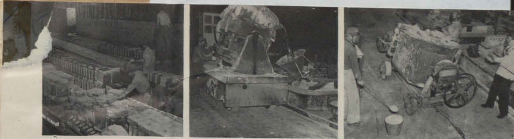
Left to right. 7—Cakes of raw materials after being conveyed from oven kilns. From here they are conveyed to crushers which break them into small pellets, which go to chlorinators where magnesium oxide is transformed into magnesium chloride. 8—From chlorinators molten magnesium chloride is carried in electrical jeeps and poured into cells. In cells are other chlorides. Direct current of high amperage, low voltage, passes through. Electro-chemical action causes metallic magnesium to rise to surface, while chlorine passes out to be re-used in process. 9—From electrolytic cells metallic magnesium is skimmed from top and poured into pots. Worker at left is ready to sprinkle flux in pot in case molten magnesium catches fire. There are 880 of these cells at Basic plant, in operation 24 hours a day, 7 days a week.
