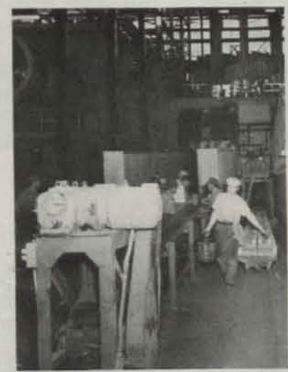
Construction view of Harrop ceramic dryer conveyor (Link-Belt) for handling green brick on edge through kiln for dehydration. Harrop kilns and dryers were used extensively in this construction.
