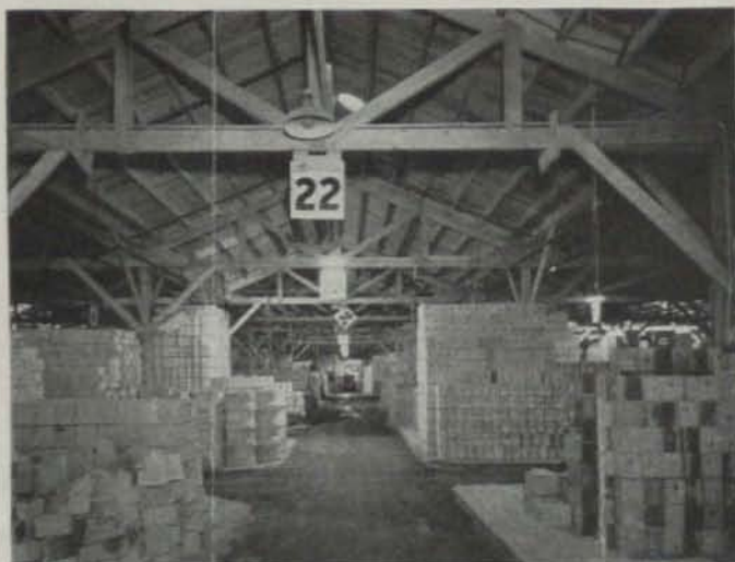
This temporary shed was constructed to stock the firebrick shapes. Large aisle in the shed made it possible to use trucks for the delivery of brick to the stock pile.
