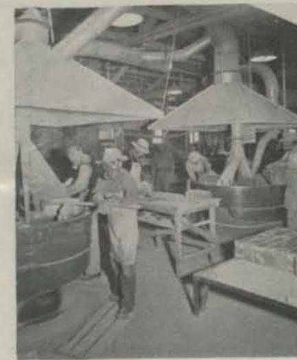
Special silicate cements were needed for the construction of the Basic Magnesium plant in Las Vegas, Nev. To avoid rapid setting, the cements were placed in V shaped pans of ice,—115 carloads of ice were used. Firebrick were ground to shape on flat grinding wheels.
