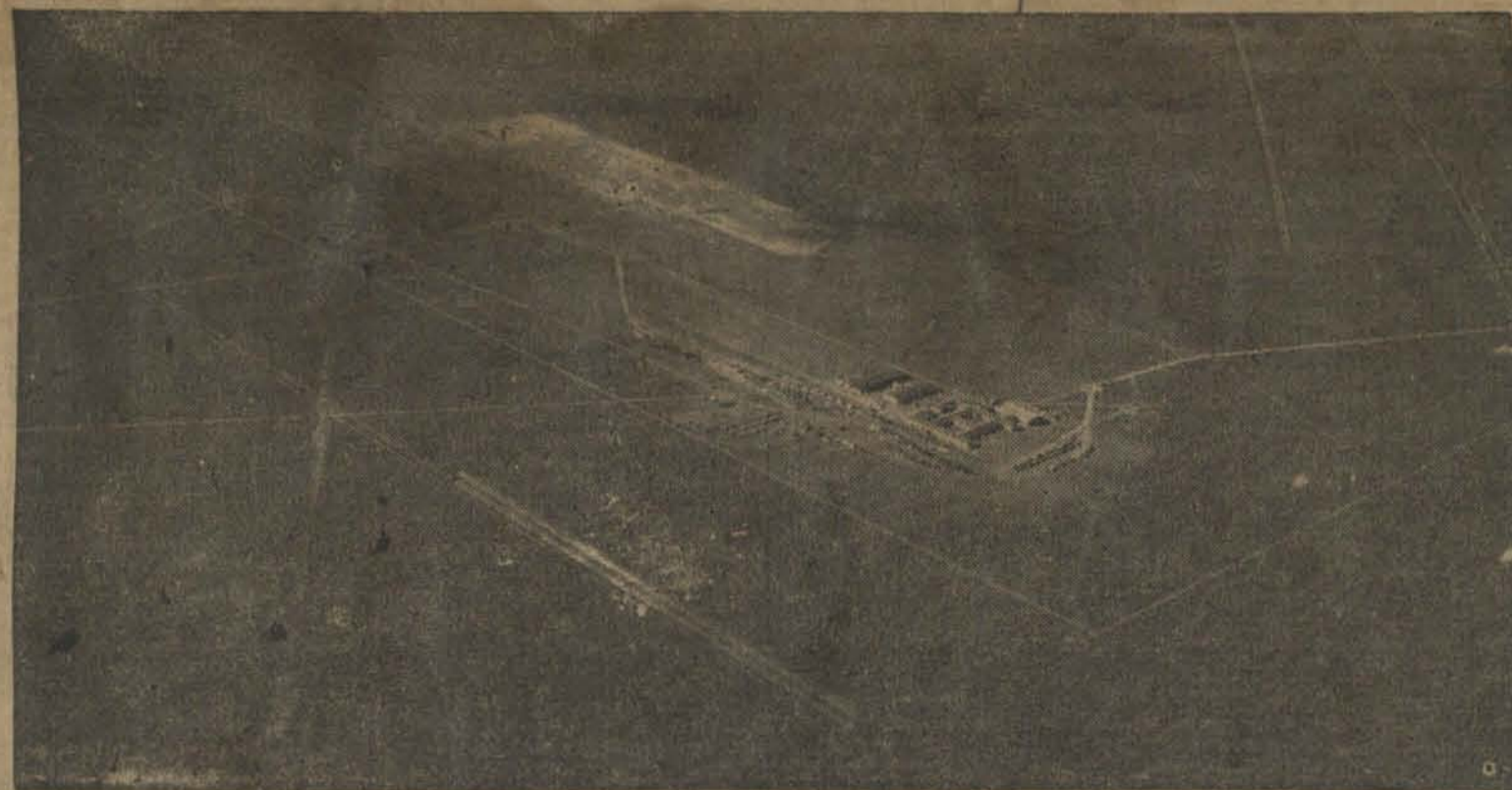
Above is shown an aerial view of the work now being done at the Basic Magnesium plant south of Las Vegas. In the center of the photograph is shown the buildings already completed at the plant, with the office building of the Basic Magnesium and McNeil Construction company the H shaped structure. To the left are seen two warehouses and the spots huddled around the buildings are automobiles. To the left and above is shown the clearing for the magnesium plant, which is going ahead rapidly. The light strip in the left foreground is a dike to protect the plant from floods, while the rectangular white line running from the left top of the picture and around the buildings is a fence. The road, leading to the Boulder highway can be seen leading from the group of buildings in the center. The dark strip across the right hand corner of the picture is the highway leading toward Las Vegas. The other white lines in the photo are roads.
