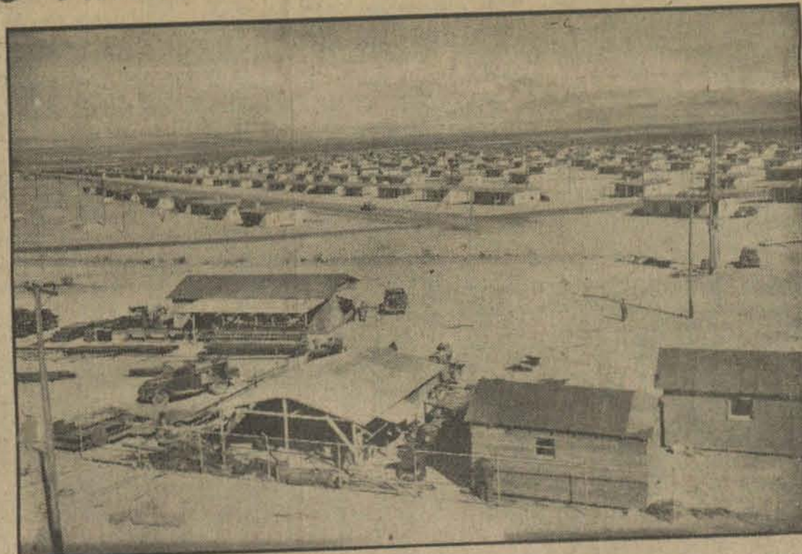
Here's a general view of a portion of the 1000 homes erected on the desert for workers at the $100,000,000 magnesium plant in southern Nevada.
