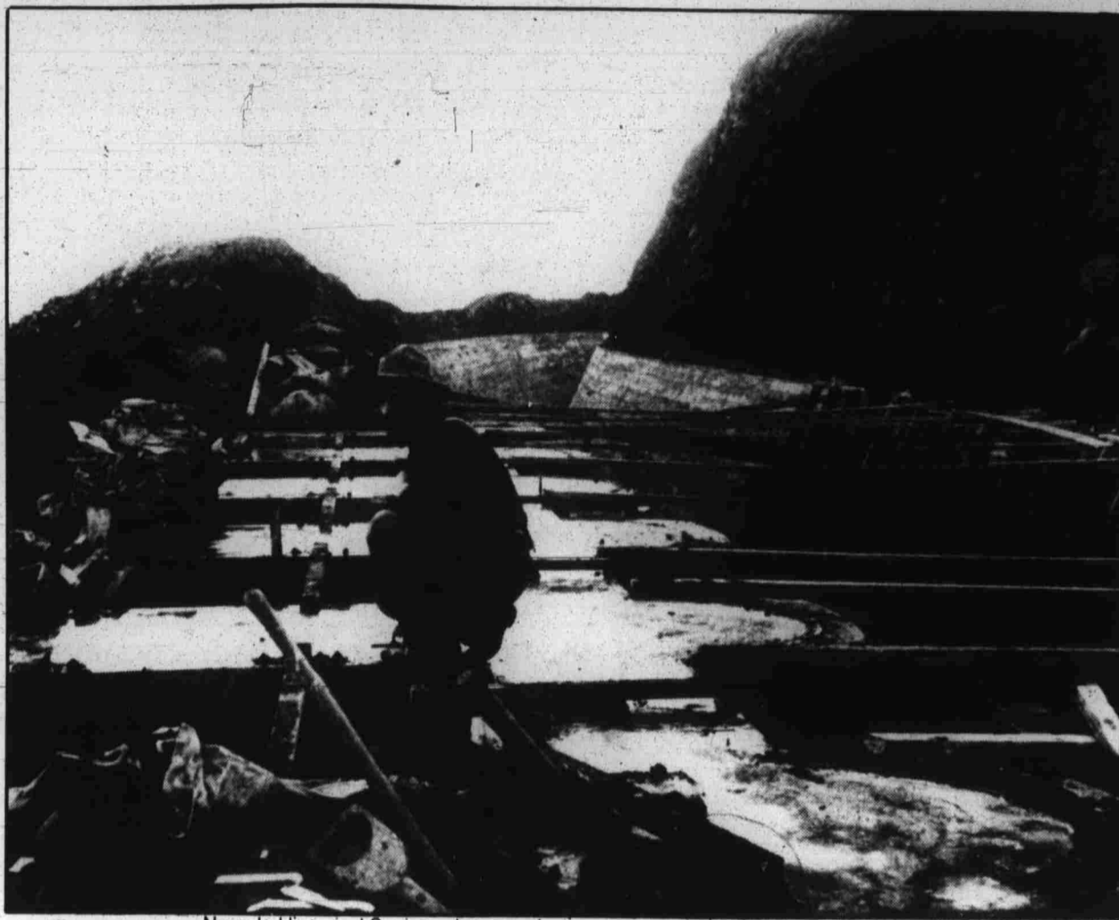
Nevada Historical Society photograph Men at work on the Truckee Canal near Derby, January 1905
