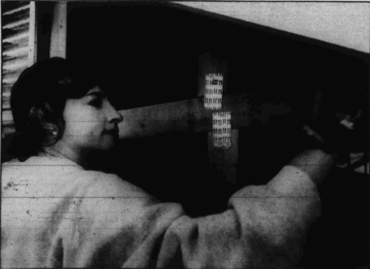
Joni Ashcraft paints the trim on the roof of her future home.
