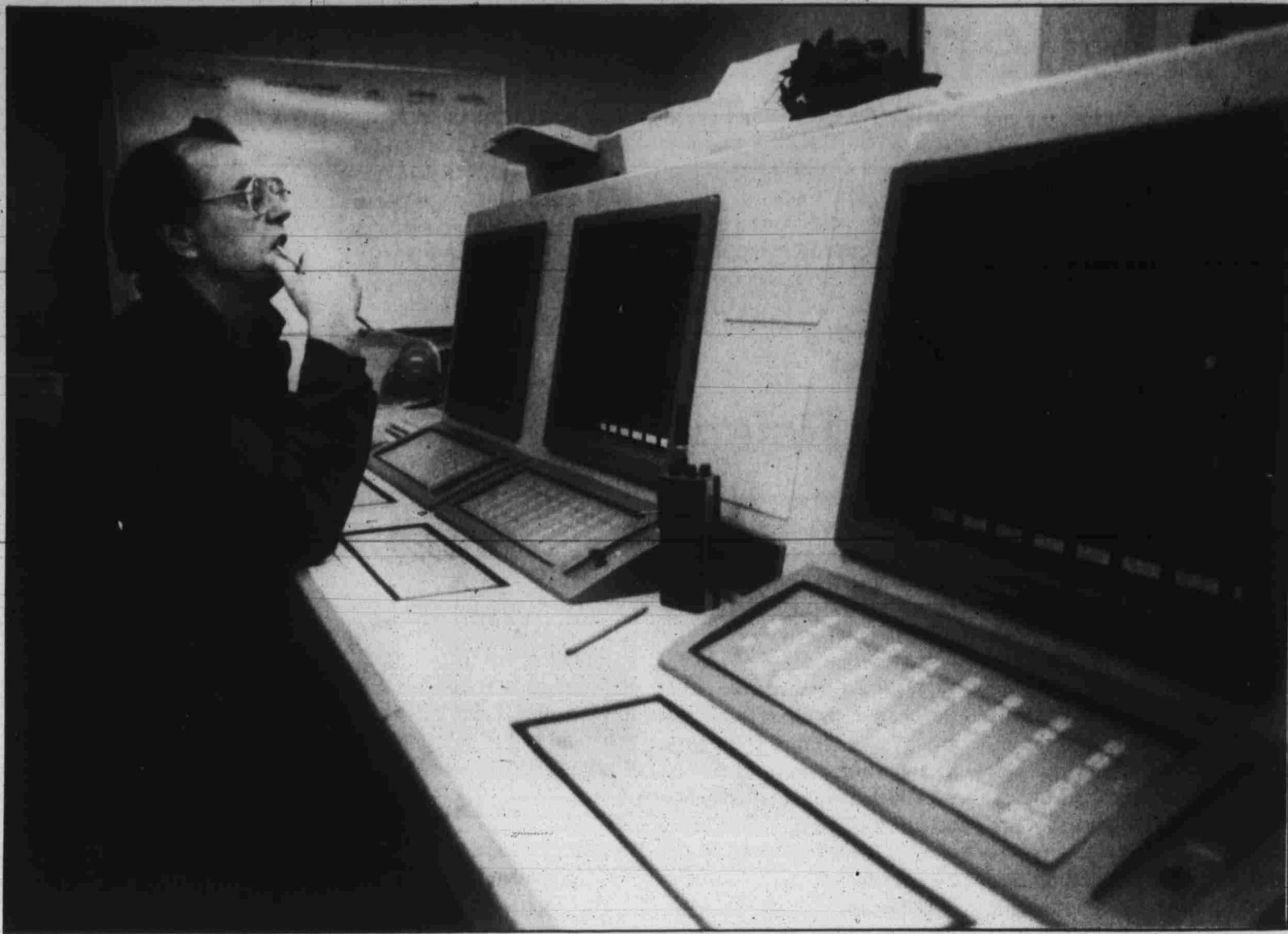
MONITORING — Delton Lyon, a senior process engineer in the sponge business unit at the Timet plant, views a computer screen at the plant. The screen enables Lyon to track the process of making titanium sponge which Timet turns into titanium ingots. Photo by Brian Jones
