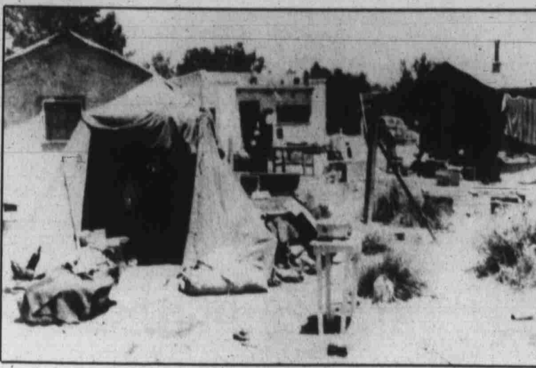
Typical housing in Westside during World War II. Photo courtesy of the Henderson Public Library
