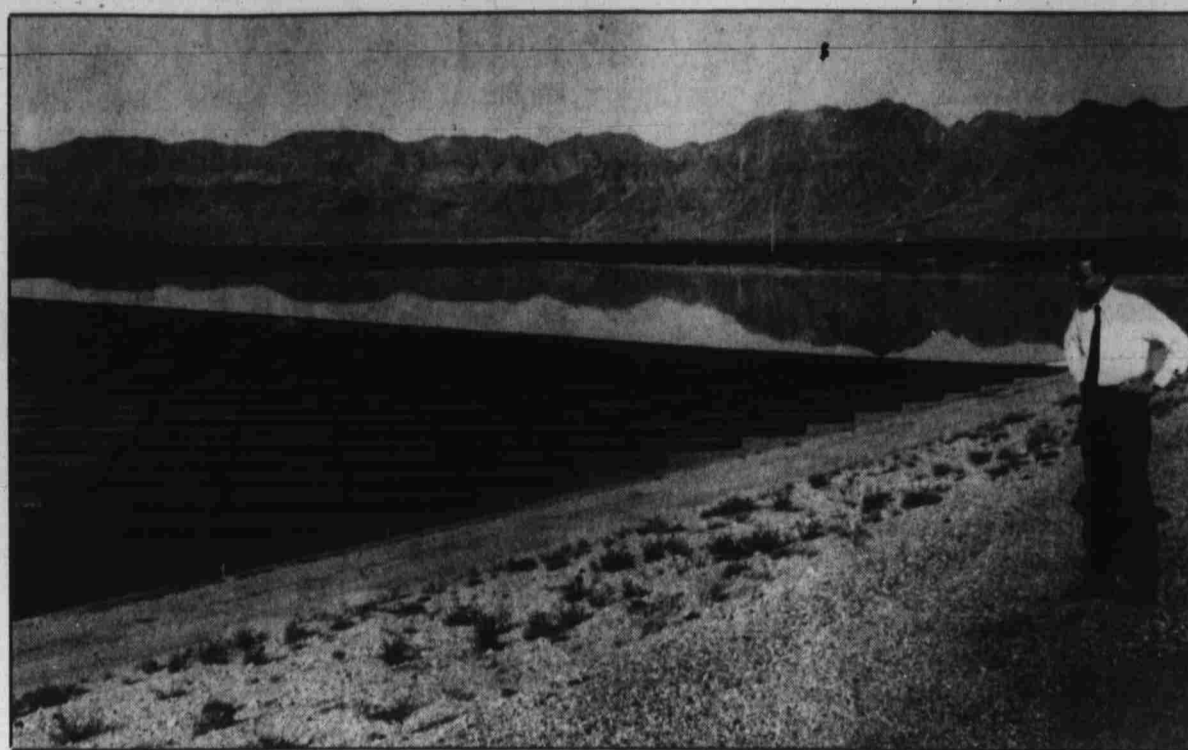
NATURAL TREATMENT—Lemna Corp.'s President and Chief Executive Officer Viet Ngo inspects the Boulder City Wastewater Treatment Facility.
