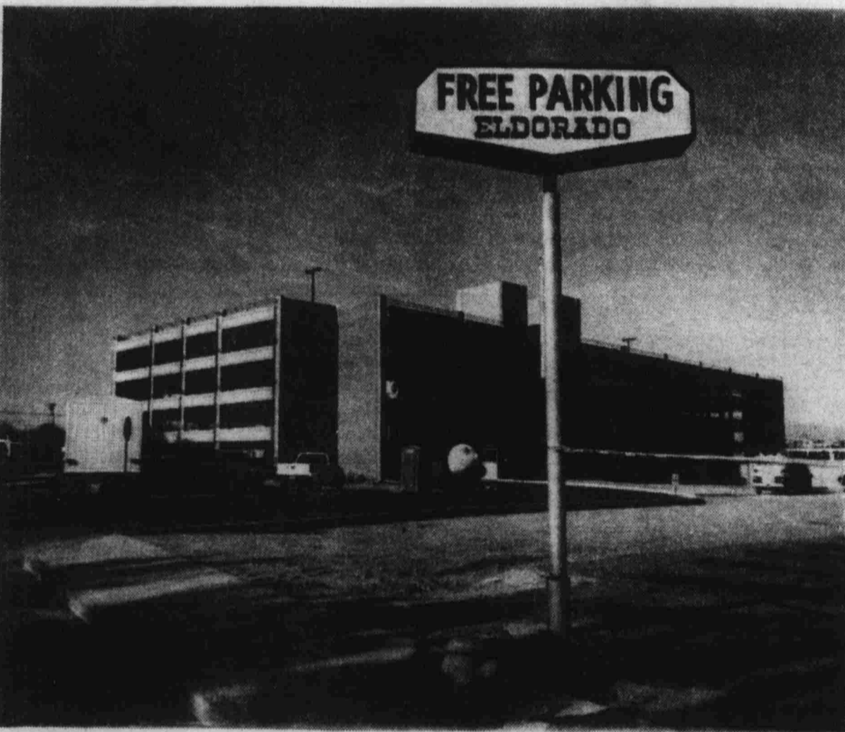
FREE PARKING —The 511-space parking garage opened recently by the Eldorado Casino features free, 24-hour, lighted park-
