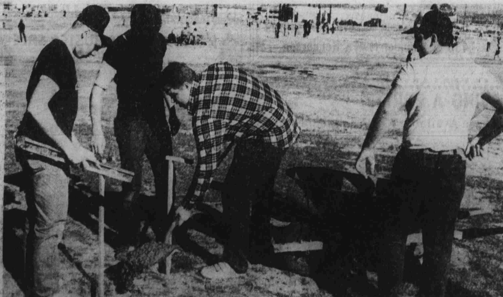
Cadets work to fill holes with concrete
