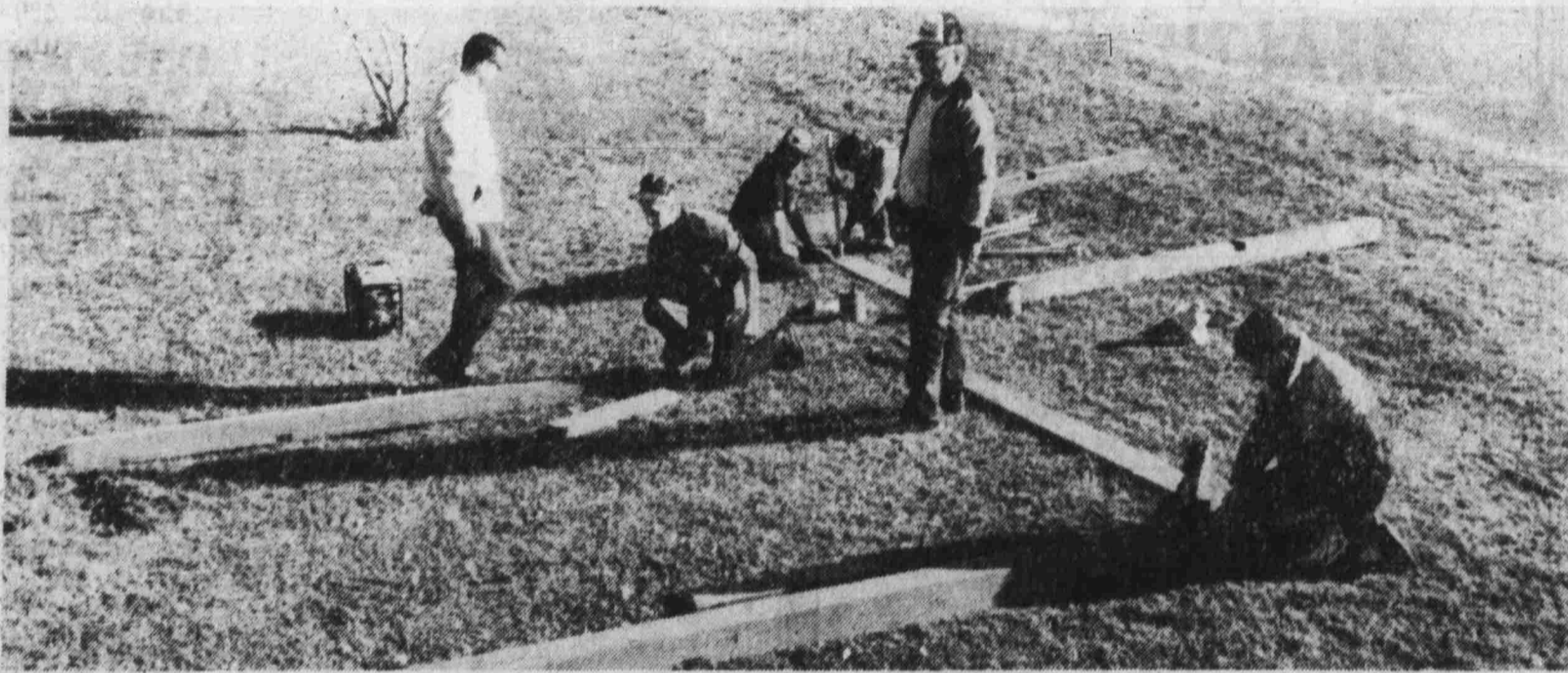
Equipment must also be assembled.
