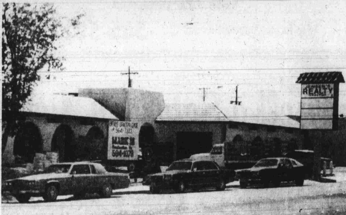
JENSEN REALTY EXPANDS— The Jensen Realty office on Water Street, near city hall, has more than doubled in size from the original Townsite house. The new construction is being done by Mark III Construction Co. The attractive Spanish type architecture makes a beautiful addition to Water Street.
