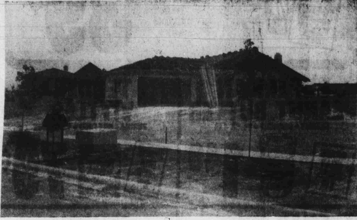
QUAIL RIDGE ESTATES CONSTRUCTION—Shown above are some of the elegant homes being built in Quail Ridge Estates in Green Valley, a luxury custom homesite development featuring 105 half acre or larger luxurious lots. During the past year housing construction has doubled in the development, with sales reaching the 43 percent mark.
