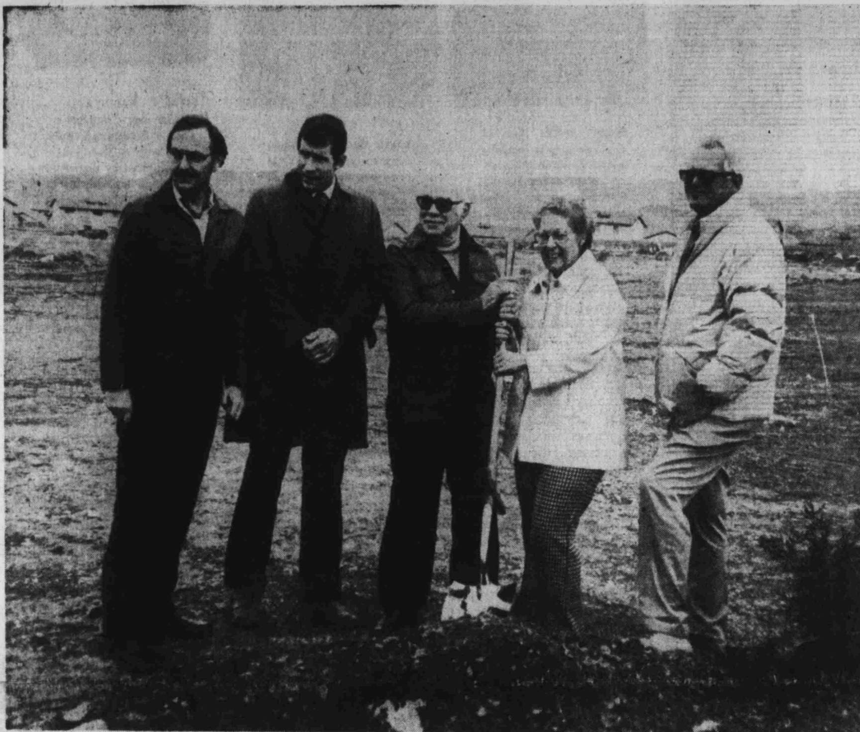
WORK TO BEGIN ON NEW ELEMENTARY SCHOOL - Ground was broken yesterday for the new Fay E. Galloway Elementary School to be located behind O'Callaghan Park. Shown above are Dr. Charles Neely, assistant director of facilities for the Clark County School District; Dundee Jones, city parks and recreation dept. director;
