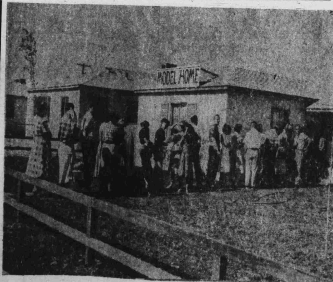
FREEDOM HOMES --- Besides the Townsite homes there were none in Henderson and when the Freedom Homes came along they were sold out in no time. They were popular as this photo indicates.
