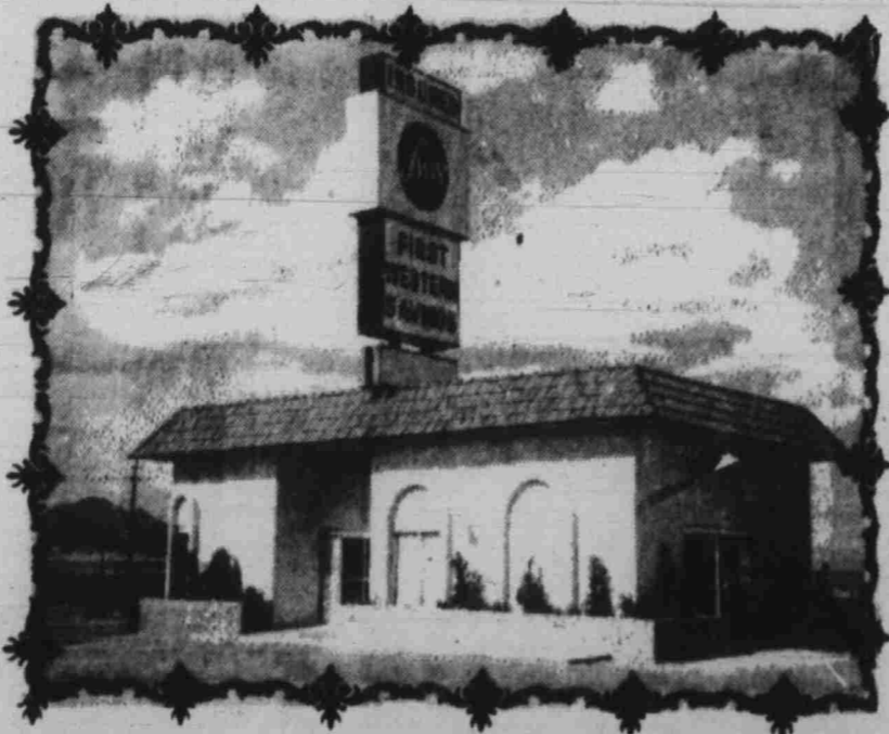
The Newly Remodeled Henderson Office of First Western Savings where you'll find complete financial services, friendly personnel, and the highest interest paid by any savings and loan in Nevada, higher than any bank.
