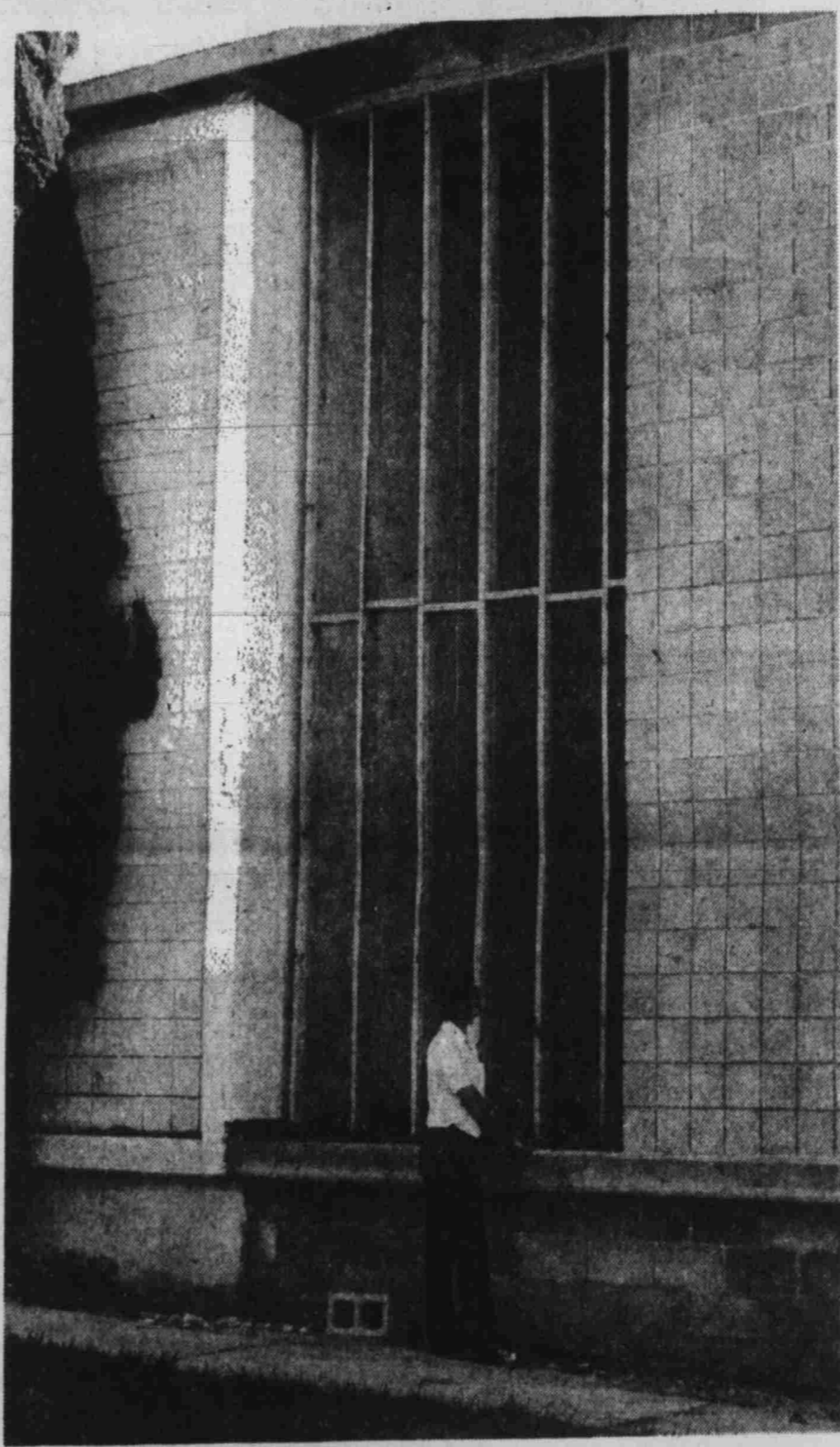
MAKING PROGRESS -- Cental Supervisor Dale Raynor examines progress on a 1,200 square foot addition to the company's Boulder City central office. The facility, which is used to connect Boulder City customers with the nation's telephone system is being expanded to make room for electronic switching equipment. The $2 million project will provide Boulder City residents with faster and more accurate connections.
