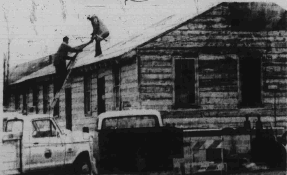
THIS WAS THE SCENE Monday morning when firemen were called to fight a blaze at the old City Hall which now serves as storage
