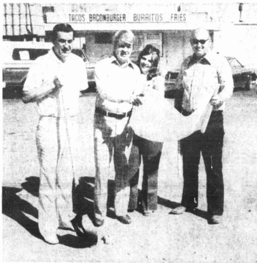
GROUND BROKEN FOR CHILDREN'S STORE--Ground was broken last Wednesday for a new children's store in Henderson. Shown at the ceremonies are Duane Laubach, president of the Chamber of Commerce; Mr. and Mrs. Gordon Cottrell, owners, and Michael Traasdahl, builder.
