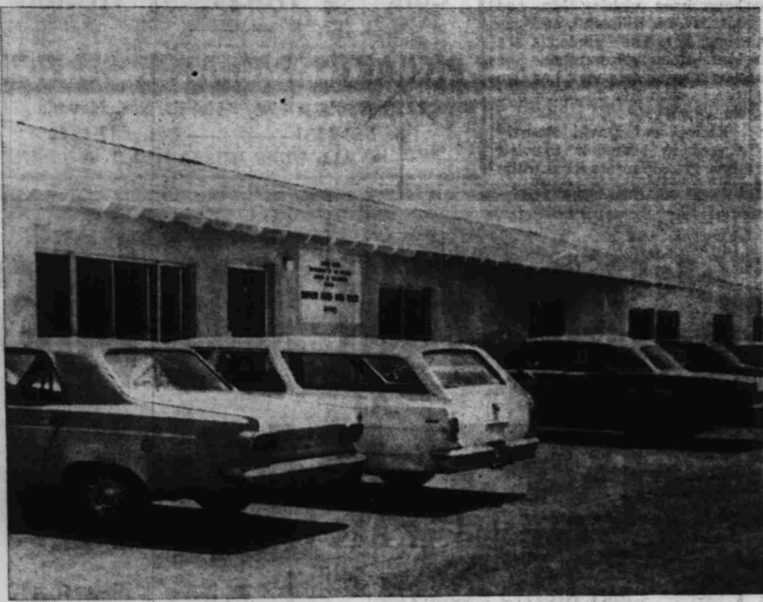
NEWEST HENDERSON OFFICE — The offices for the construction of the Southern Nevada Water Project which will bring millions of gallons more water into this area, are located on Lake Mead Drive where a building for that purpose was constructed. Henderson was selected as a central site for the project, headquarters. Around 40 employees are working in this office now, and there will eventually be around 100.
