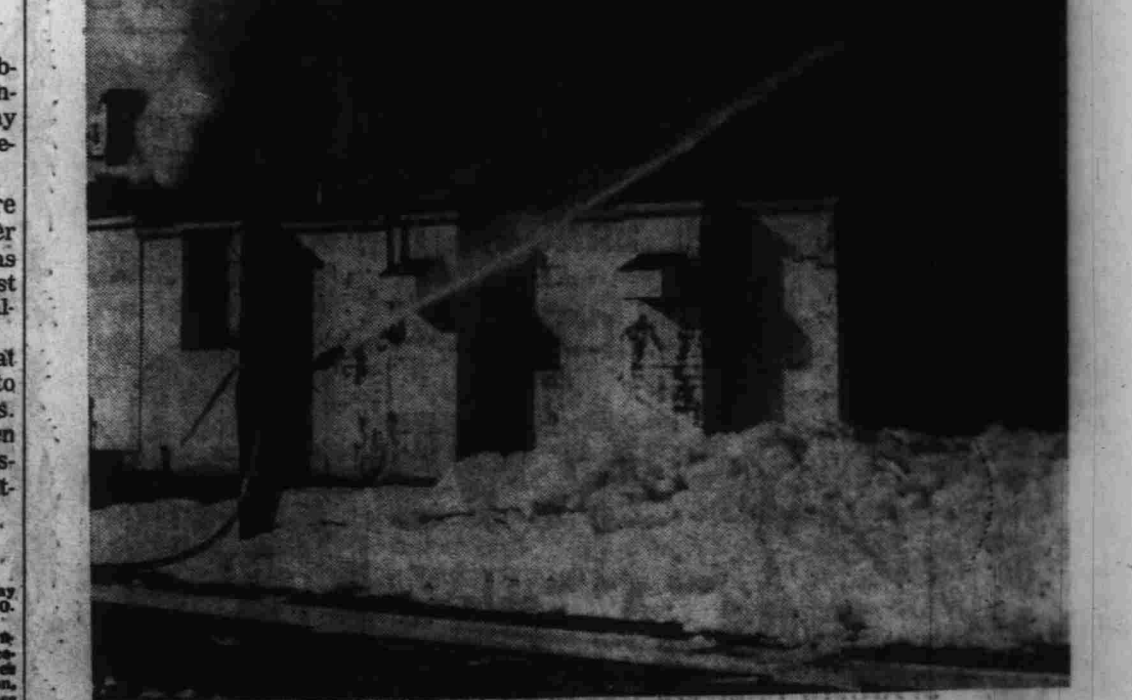
FIRE DEMONSTRATION — Old Administration buildings at American Potash and Chemical Corp. were burned last Friday during a fire demonstration. What looks like snow in the foreground is High X foam put out by the Kibbie Co which was used in the demonstration. Firemen kept the blaze under control as the old buildings were demolished.
