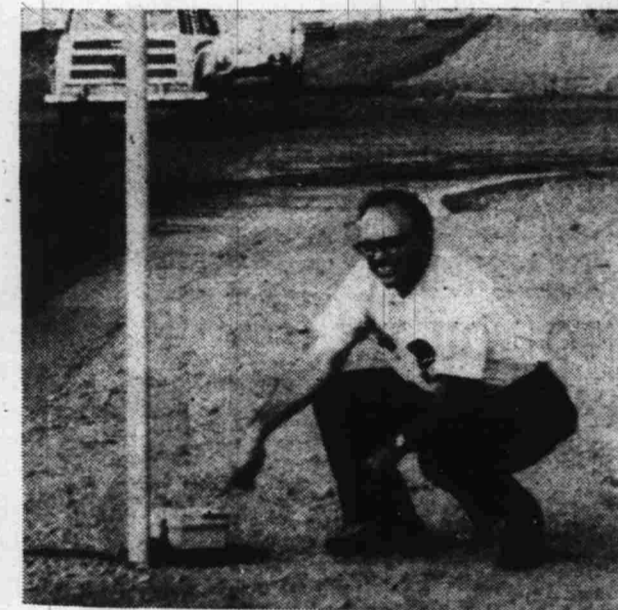
NOT ATTRACTIVE — Two years ago with the prodding of Assemblyman Gibson, work was started on a four-lane highway through Henderson toward Lake Mead.
