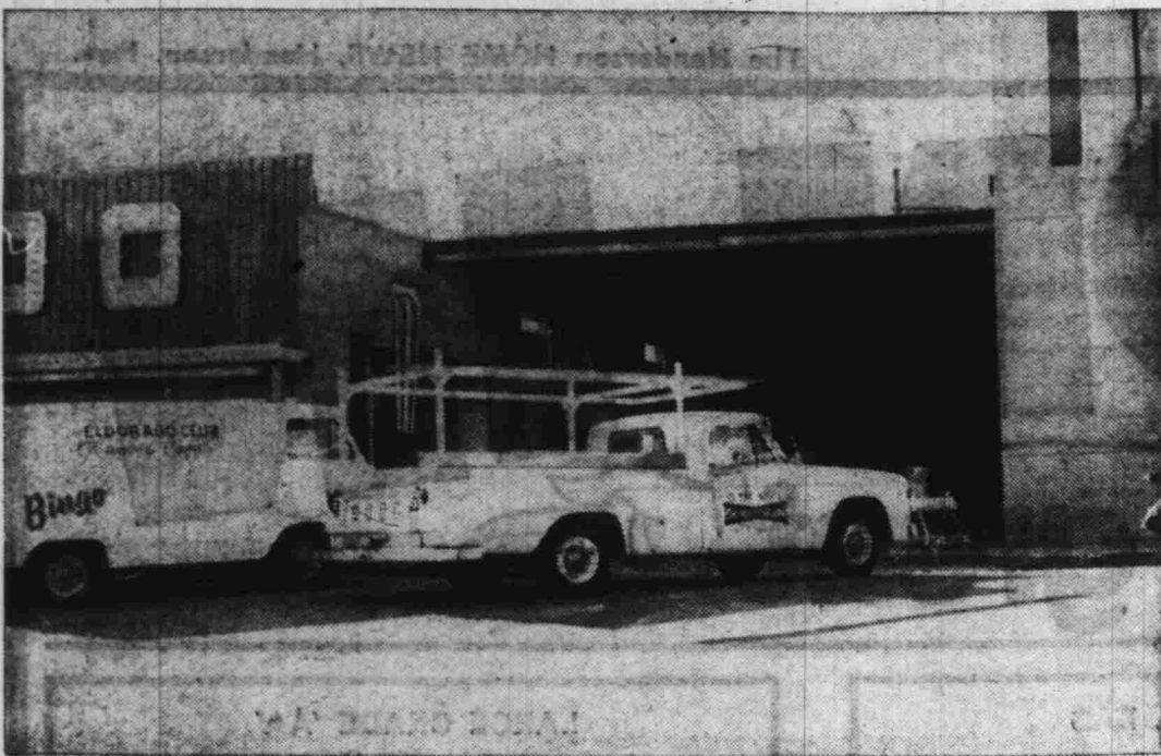
BUILDINGS JOINED — Construction at the Eldorado Club has now reached a point where the Eldorado and the former Royal Club have been joined across the former alley at the first floor level and the sidewalk is cleared of construction machinery. Partitions have been removed from the former Royal premises to make way for remodeling of the building and installation of new facilities of the Eldorado Club.
