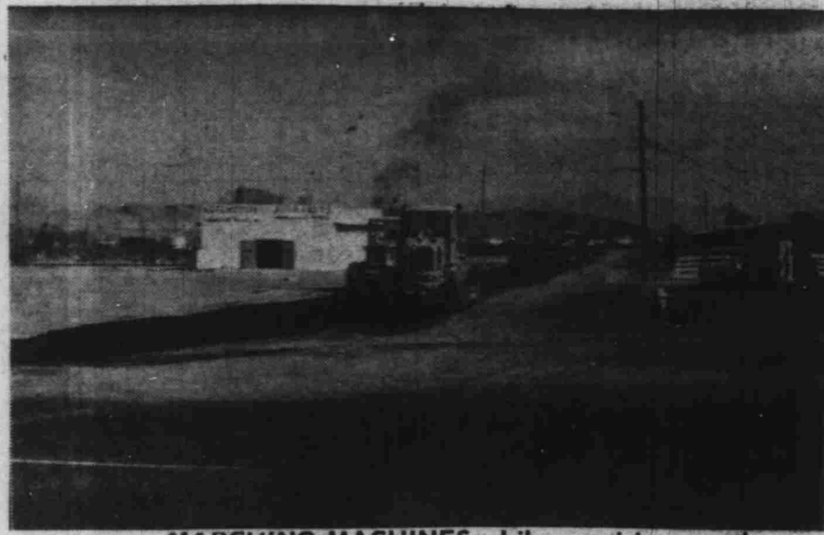
MARCHING MACHINES —Like precision marchers the graders promenade down Moser and Corn street as they turn this long heap of oil and gravel to the left then to the right for thorough mixing.
