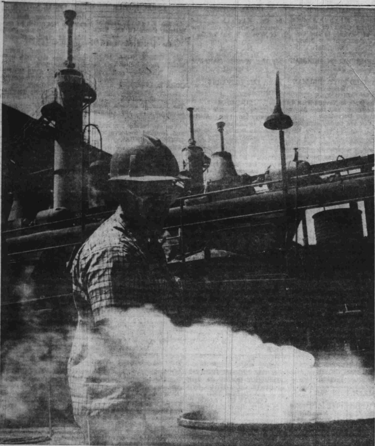
SKY WRITER'S DREAM —Smoke pouring from a four-ounce sample of titanium tetrachloride shows why sky writers have adopted this material for the messages they emblazon in the air. This product is generated in production of titanium metal. To prevent it from escaping, Titanium Metals Corporation of America has installed the equipment shown in the background of this photo a complex maze of vats, pipes and towers whose sole job is to prevent permanent messages from being smeared over Clark County skies. Smoke
