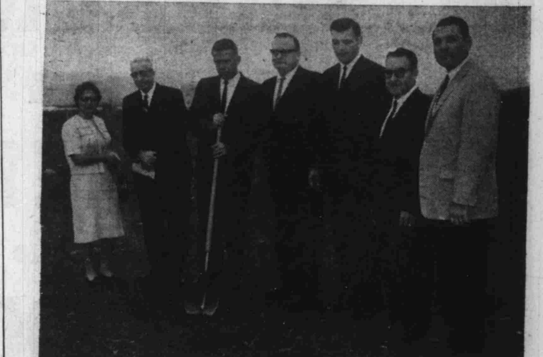
GROUND BREAKING HELD—Officials for the Palm Mortuary are shown breaking ground for a new $300,000 Henderson Mortuary and Mausoleum on Boulder Highway. Construction was set to begin Monday. Shown, from left, are Selma Bartlett, Henderson manager of the Bank of Nevada; Reverend Ford T. Gilbert, general manager of the new mortuary; Charles Knauss, Jerry Woodbury, Dallas Brossard, co-owners with Don DeVoe, and Lou LaPorta, county commission chairman.
