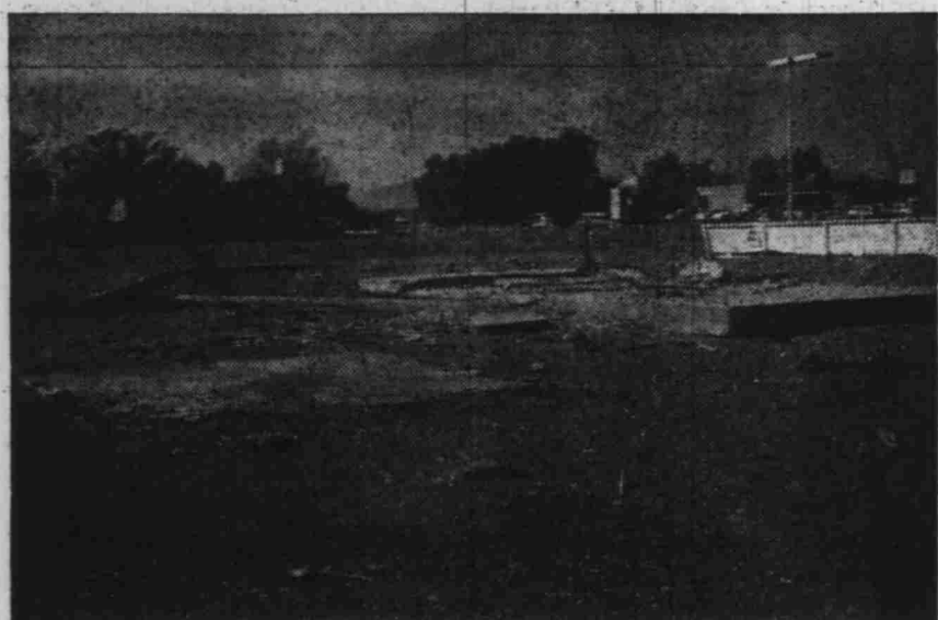
ON BOULDER HIGHWAY — This mess is the remains of the old Loveland Market which was condemned and torn down several years ago by the City in exchange for the lumber which was used in remodeling the Henderson Boys Club. It is located immediately South of the Hancock Station.
