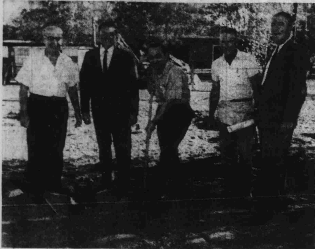
GROUND BREAKING —Herb Crosby turns the first spade of earth at ground breaking ceremonies marking the start of construction of a modern two story building at 19 Water Street which will house the Crosby Music Center, three other stores and four apartments. Watching, from left, are Mayor Bill Byrne, County Commissioner Lou F. La Porta, Construction Superintendent A. V. Geier and R. Julian Moore, Vice-President of Frontier Fidelity.
