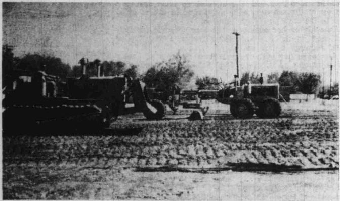
**CITY HALL SITE** — City equipment is shown working at the location of the new City Hall on Water Street across from the Townsite School. A nine-foot slope between Water Street and the alley will require approximately 12,000 cubic yards of earth to level the building site before construction starts.
