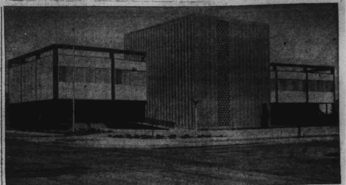
NEW ESD BUILDING — The new million-dollar home of the Nevada Employment Security Department, located at Second and Valley Streets in Carson City, was occupied this week by the agency's staff of 100. The main entrance is shown at the left, directly behind the flagpole. Features of the building include conveniently located public restrooms, an auditorium and a lounge for the employees.
