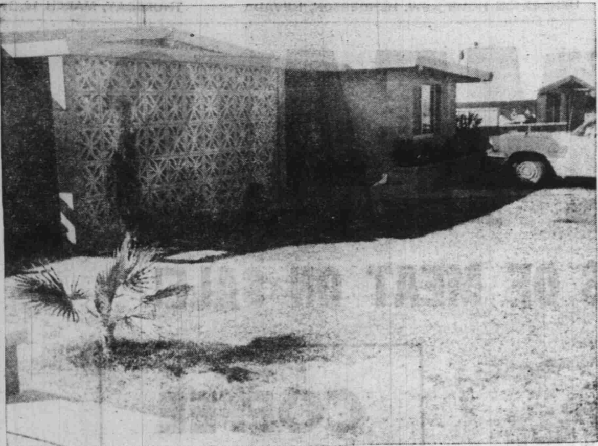
GRACEFUL AND DURABLE — The lovely, traceried patterns created by the decorator block wall on the front of the house look like lacework done by a giant hand. The delicate appearance belies the durability of these concrete blocks.
