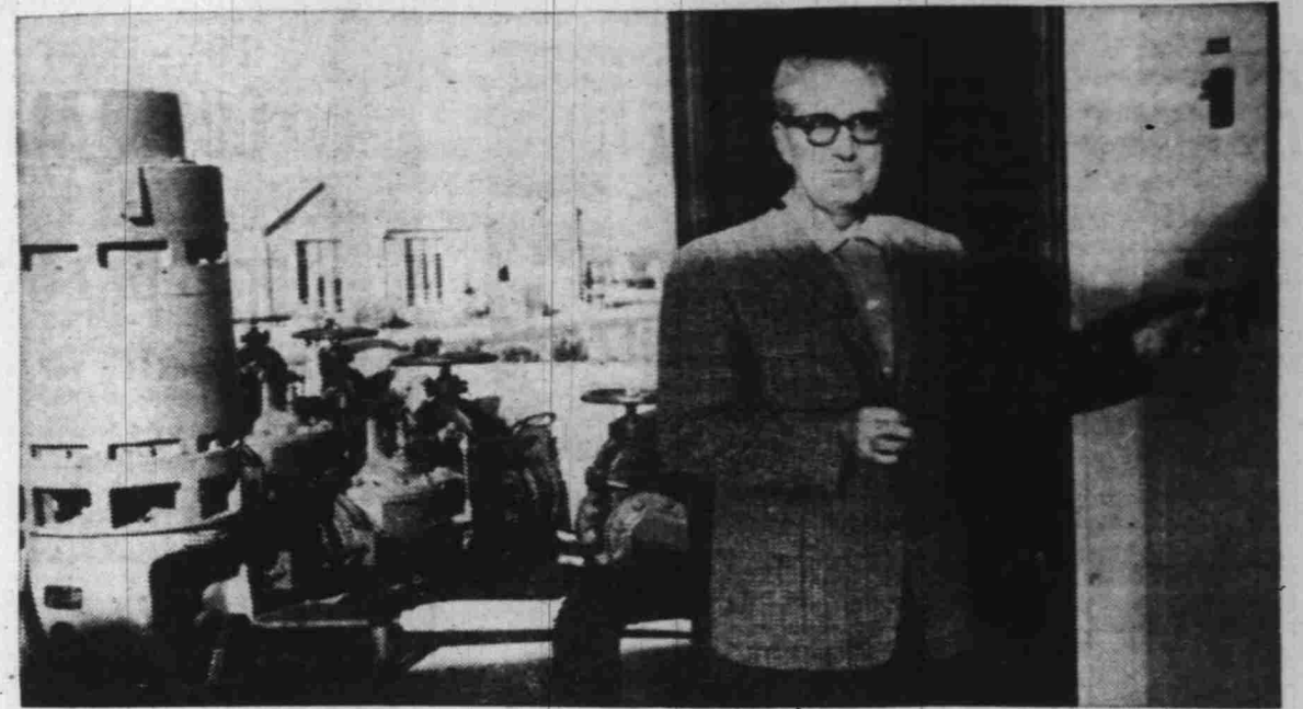
HERE COMES THE WATER — Mayor Bill Byrne pushes the button to start the pumps on the new water system recently finished. The pumps will fill the 1,500,000 gallon reservoir tank and add pressure to the upper third of the city. With increased pressure, the Fire Department will be in a better position to fight fires in the business district and homeowners will notice a much-needed increase in the pressure at house taps. This will be especially noted next summer when water usage balloons.
