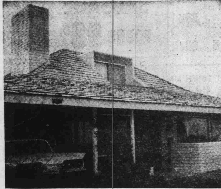
ONE OF THE FEW SUCH HOMES in the area, the Hershel Trumbo home combines traditional with modern. An English-type shaké roof, and two stories more common in the East, are combined with brick construction characteristic of Nevada buildings. Architect Jack Miller helped remodel it and give this home its present distinctive style.
