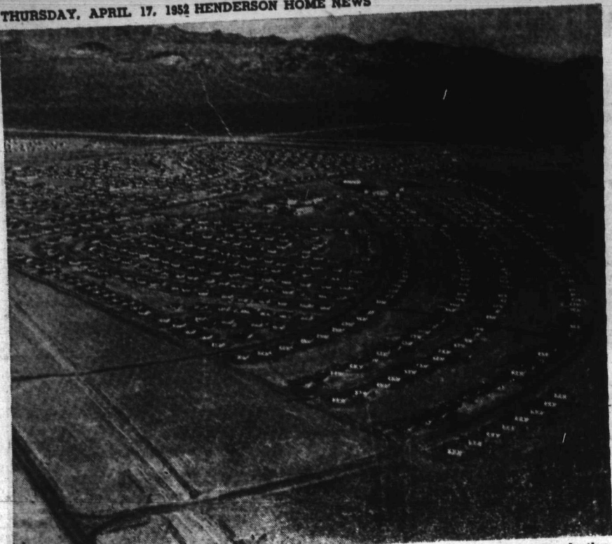
Shown above is an aerial view of the Henderson Townsite in the early days of plant production. The picture is still the same, if it were taken to-day, except for the addition of plentiful trees, more store buildings and now the 350 more newhouses being constructed by Federal Homes Development Co.
