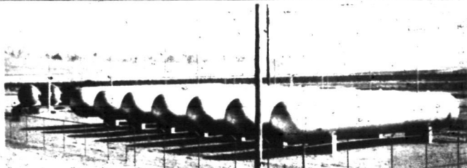
These storage tanks held thousands of cubic feet of propane gas which, under high pressure, was piped to BMI refineries for furnaces which heated crucibles. Noted for fantastic equipment, BMI was supplied with liquid propane gas in metal ball tank trucks, one of which may be observed in the background. Coated with aluminum paint (because magnesium paint has not yet been marketed) these storage tanks were a landmark at the world's largest magnesium plant.
