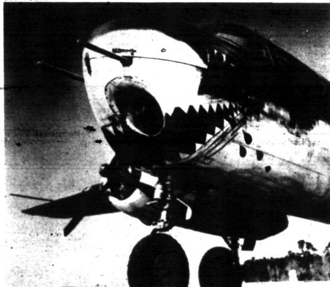
This Sky Shark is a B-25 Mitchell medium bomber. Picture of the business end of this sky-terror shows how the 75-mm cannon is set in the nose. Mounted above are two 50 calibre machine guns. On the upper left nose, partially hidden by a machine gun muzzle, is a camera for recording action. This plane has proved itself in combat. It has sunk ships at sea with direct hits from the cannon. These Mitchells use considerable magnesium. Several parts are made from metal produced at BMI.
