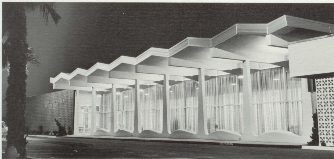
Clark County School District Education Center
