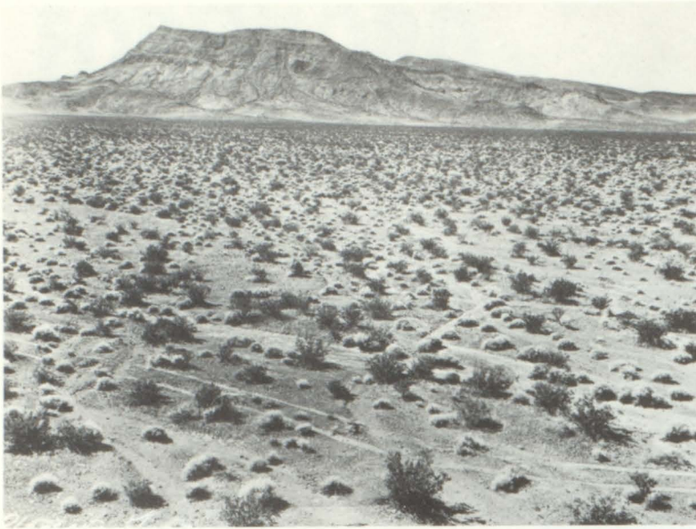
Henderson Sept. 11, 1941, just before groundbreaking
