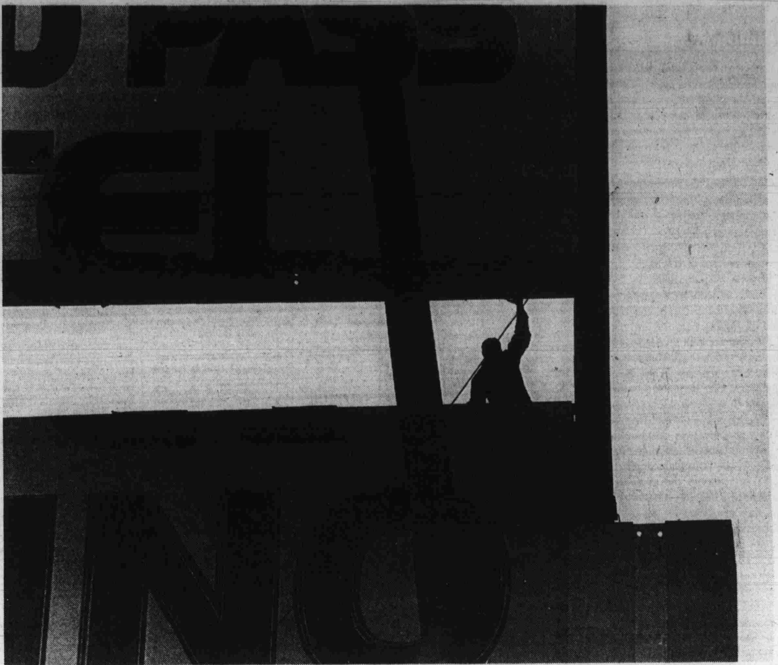
A workman is silhouetted by morning light as the Railroad Pass Hotel and Casino sign is completed
