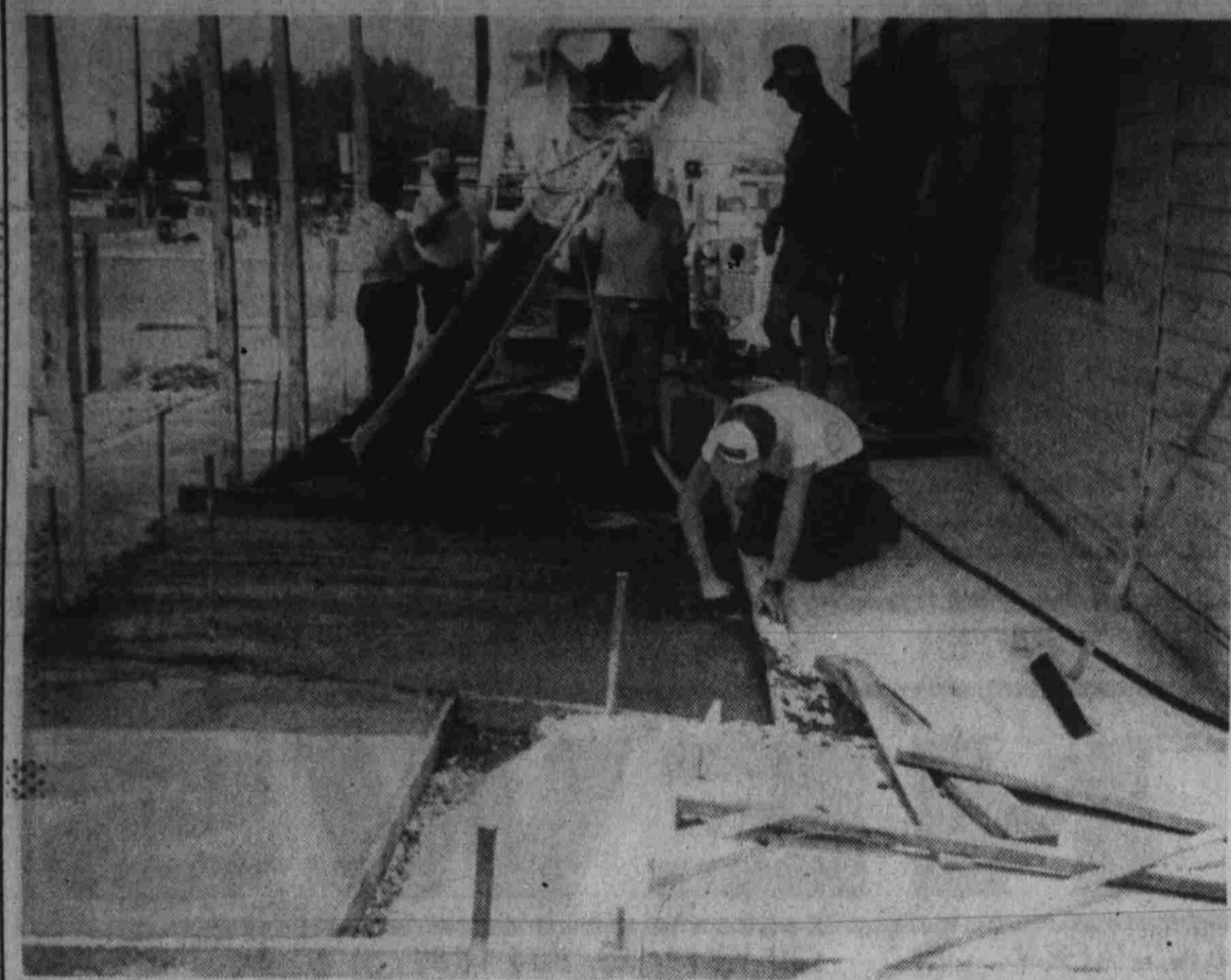
KIWANIANS BUILD WHEELCHAIR RUNWAY —Members of the Henderson Kiwanis Club completed building a concrete runway at the home of Jim Heller at 306 Water St. The runway will assist Heller in entering and leaving his residence in his wheelchair. Due to the generosity of Basic Ready Mix, who donated the concrete, the Kiwanians were able to also construct a small patio at the same time, which Heller intends to utilize for entertaining with his many friends. Members assisting on the project were John Freels, Bill Giles, John McDevitt, Rex Newell, Delwin Potter, Tom Ryan and Jim Thomas.
